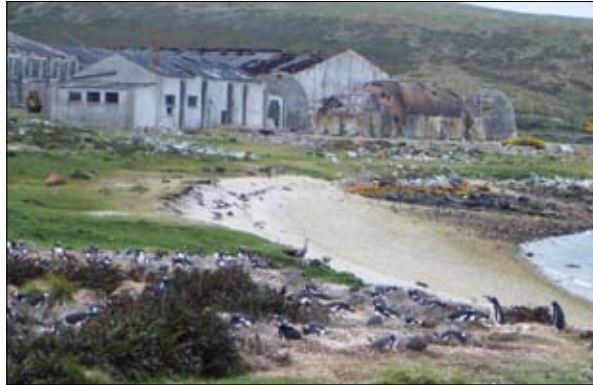
Disused and subsequently bombed mutton processing plant at Ajax Bay, San Carlos Water. This became the forward dressing station, the "Red and Green Life Machine" during the Falklands War.
